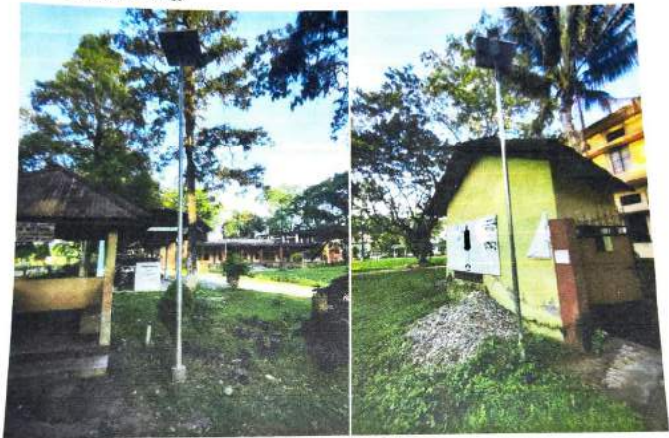
Fig.-7: Solar street lamps
